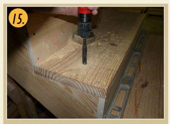
Drill a 1/2" hole into the tread, knee wall, or landing tread. Also, drill a 1 1/2" deep hole into the underside of the handrail.
