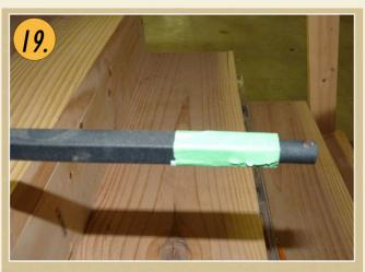
Apply painters tape around the top of the balusters before installing (not covering the round portion of the baluster).
