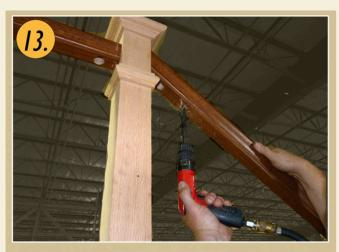
Whether you are doing new installation, or replacing old balusters, you need to ensure you have holes at the appropriate sizes and depths.
