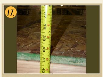
Measure the distance from the bottom of the handrail to the top of the tread or knee wall.
