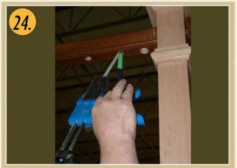
Apply a little more epoxy into both the top and bottom hole. The tape provides a barrier so that any epoxy that comes out of the hole will stick to the tape instead of the baluster.
