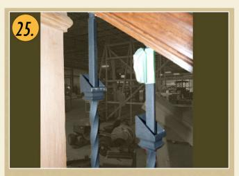
Allow the balusters to sit for up to 24 hours before removing the tape and fastening the shoes.
