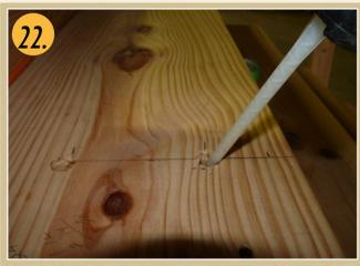
Fill 25% - 40% of each hole (top and bottom) with epoxy. The epoxy Stair Supplies sells is thicker than most, so it won't be as likely to drip.
