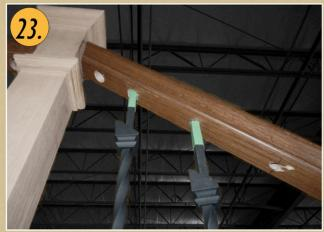
Once you cut your balusters to length, slide them up into the handrail, and then drop them into the bottom hole. Make sure they are straight and any angled shoes are facing the correct direction.
