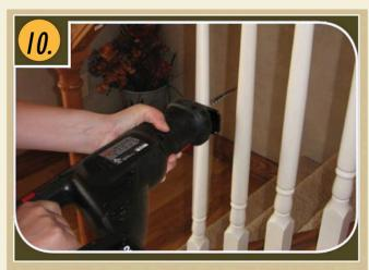
If you are replacing wood balusters, cut in the middle to remove the old balusters.
