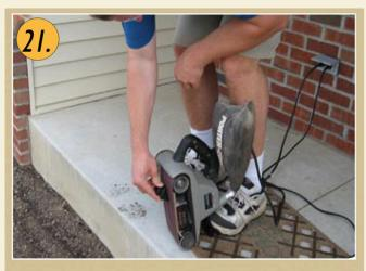
Angled shoes are designed to work with 90% of stairways. For the other 10% the angle can be adjusted using a belt sander for a perfect fit.
