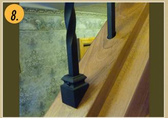
Bottom shoes are recommended, while top shoes are less common. This is because the rounded portion of the top of the baluster looks more finished going into a round hole. Also it's less visible on the underside of the handrail.
