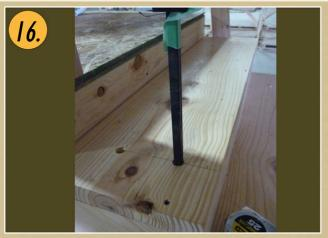
Once you have cut the balusters, this will allow you to slide the baluster up into the handrail FIRST and then drop it down into the bottom hole.
