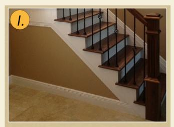
Iron balusters can be installed into Treads...
