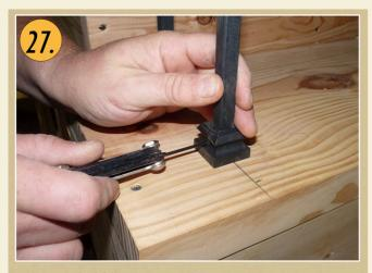
Using a 3/32" allen wrench tighten the set screw that comes pre installed in each aluminum shoe.
