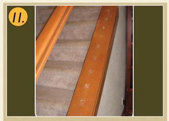
Make sure to remove all dowel screws and finishing nails from whatever surface your balusters were installed into (Knee Wall pictured).
