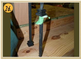
After you have waited 24 hours, remove the tape from the bottom shoes, and lower them into position.
